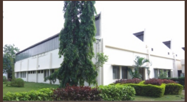
Hydraulic Pumps & Motors Plant
