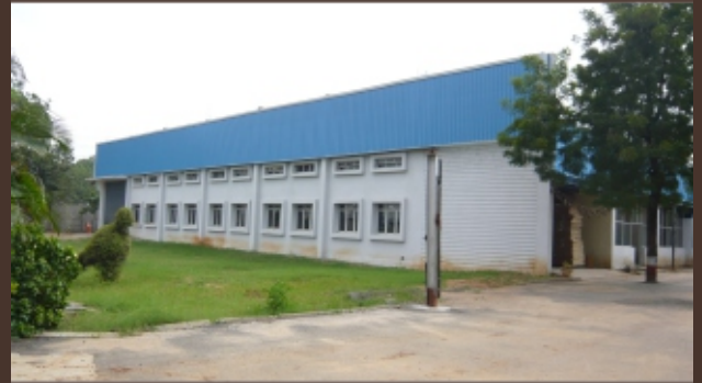
Hydraulic Valves Plant
